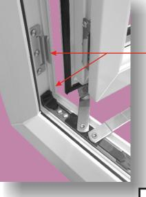
Fit Stay Guard Elite approx 75mm centres from the internal corner as show here. Secure using 4.8 X 25 carbon steel zinc coated screws
